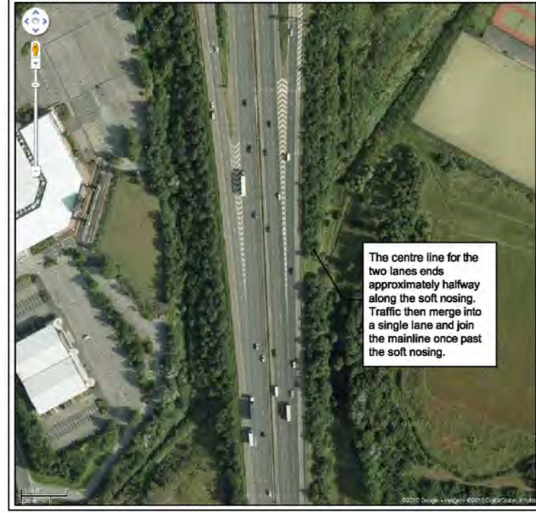
EXAMPLE OF RAMP METERING MERGE FROM TWO LANES TO ONE - M6 J10 SOUTHBOUND
